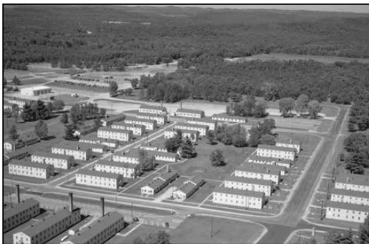
Above: 800 series buildings at Fort McCoy, Wisconsin
